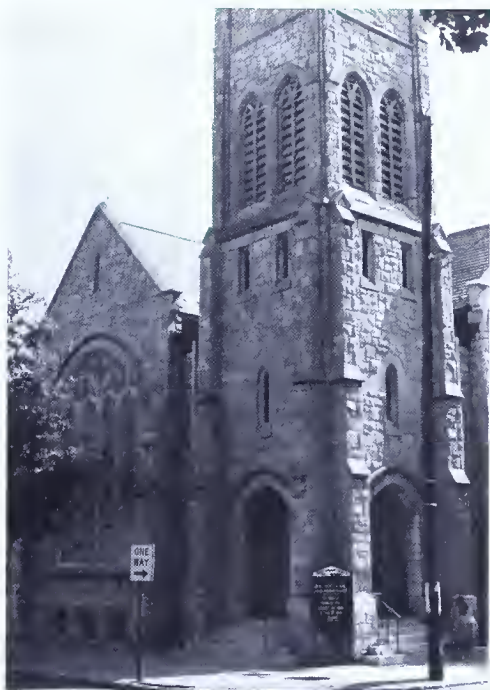
Derry Street United Methodist Church, Fifteenth and Derry Streets; Cockeysville marble from southern Chester County.
